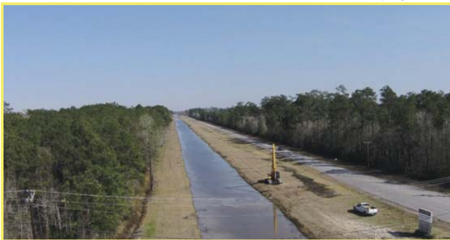
Mechanical Removal of Vegetation from the Water Supply Canal
