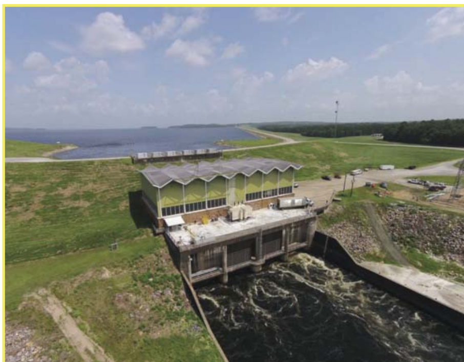
Toledo Bend Dam and Powerhouse
