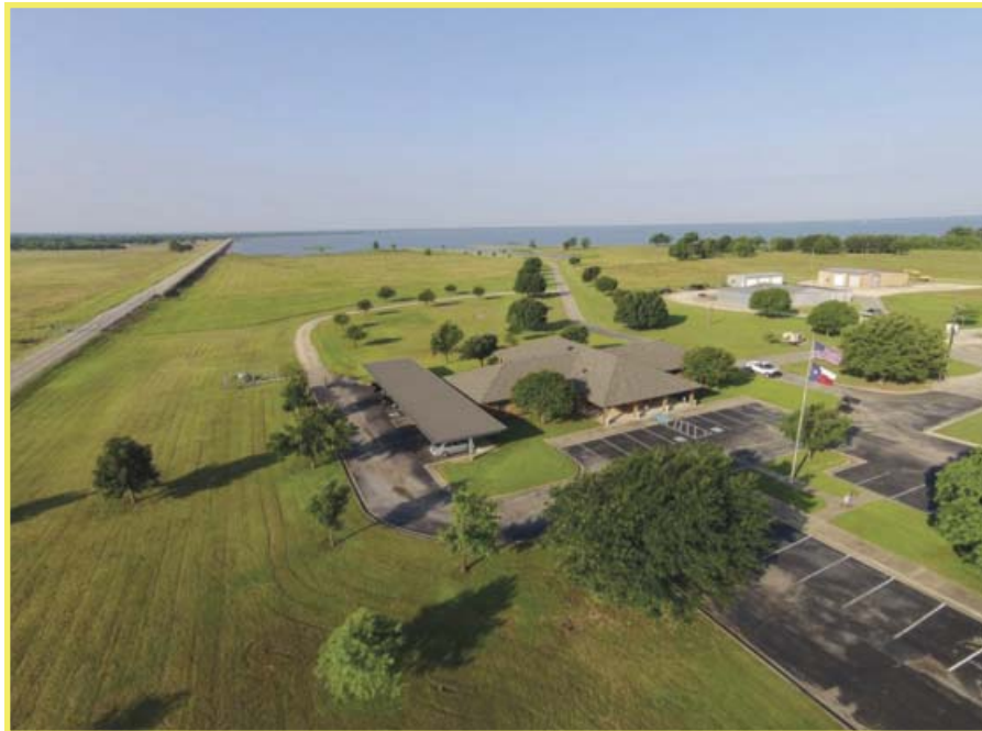
Iron Bridge Division Offices
