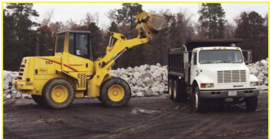
Loading Rip-Rap for Shoreline Management
