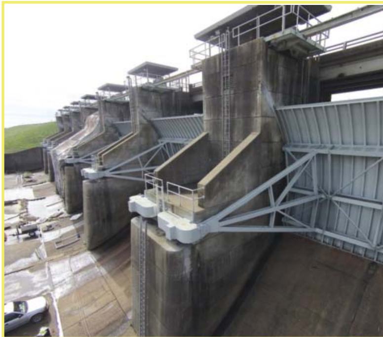
Gate Refurbishment at Toledo Bend Spillway
