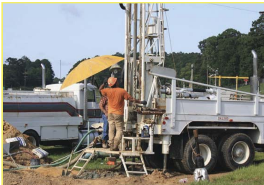
Drilling New Relief Well Near the Powerhouse
