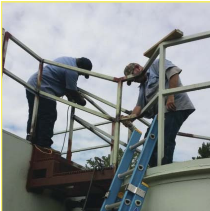
Assembling Frontier Park Wastewater Treatment Plant
