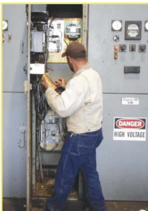
Pump Control System Maintenance
