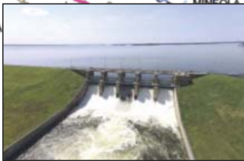
Lake Fork Dam & Reservoir
