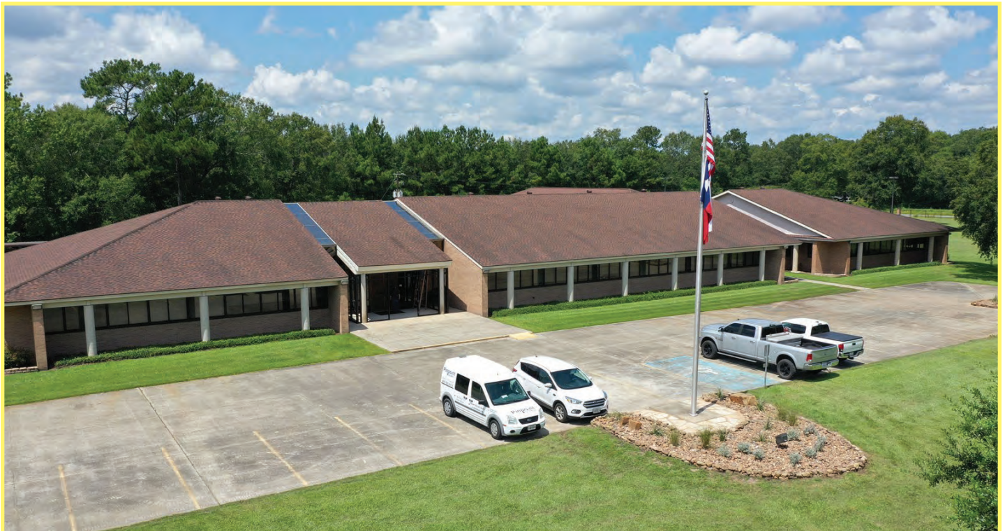
Sabine River Authority General Office
