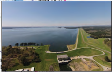
Toledo Bend Dam & Reservoir
