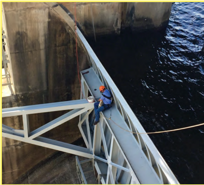
Tainter Gate Maintenance
