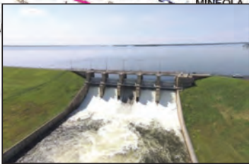
Lake Fork Dam & Reservoir
