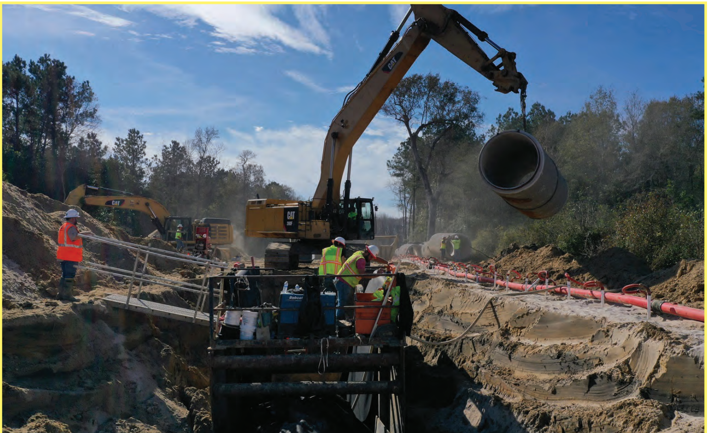
Laying 66-inch Pipe in the 7-Mile Right-of-Way
