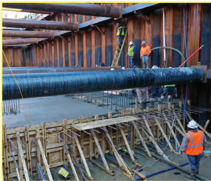
Pump Station Wet Well with Center Section Floor Being Finished
