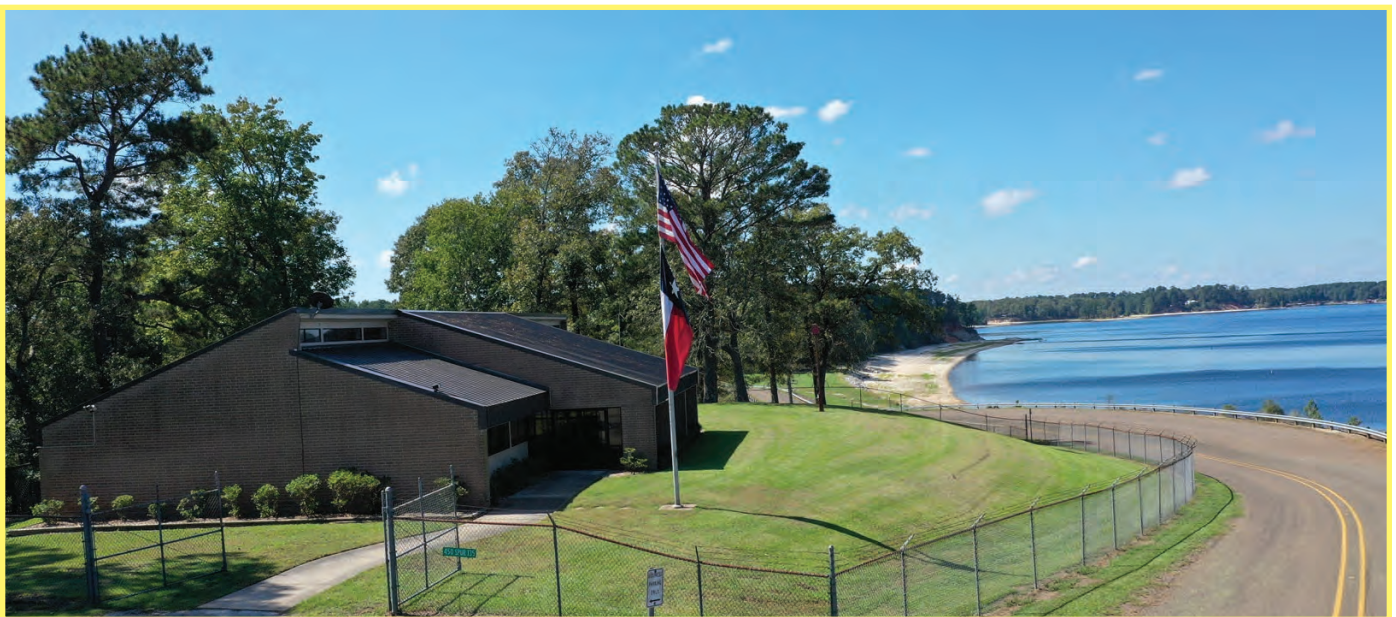
SRA, Toledo Bend Division Offices
