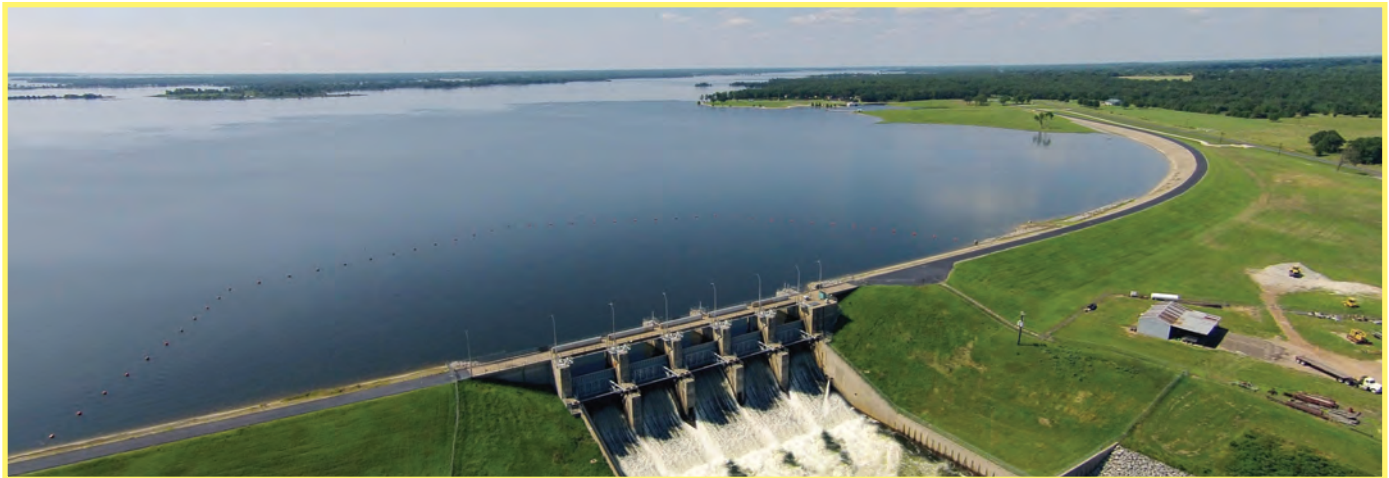
Lake Fork Dam and Reservoir
