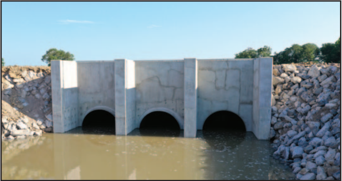
Womack Project concrete headwall complete
