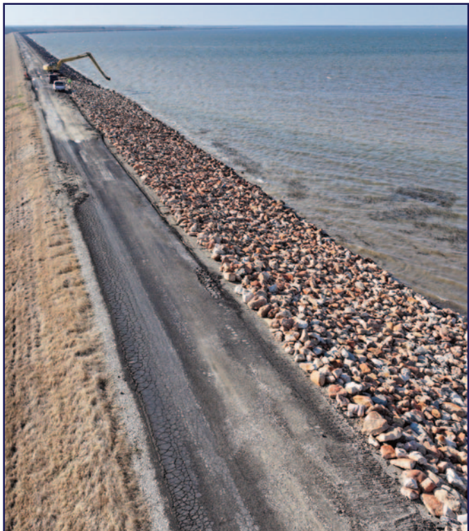
Riprap repair on the upstream face of the dam
