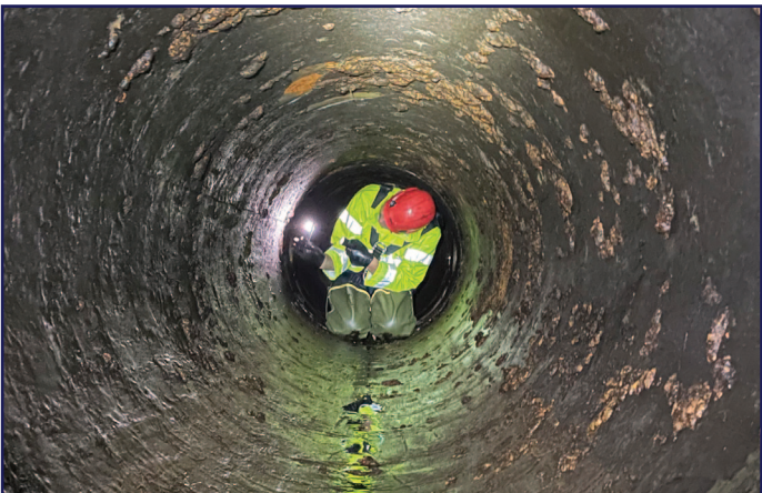
Release pipe inspection
