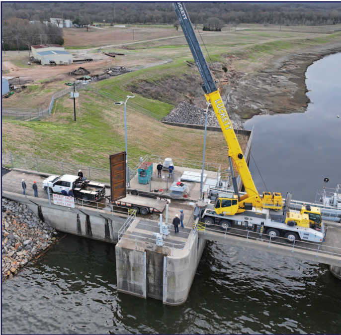
Removing bar screen for inspection
