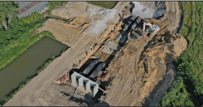
East Wynn Siphon Replacement Project
