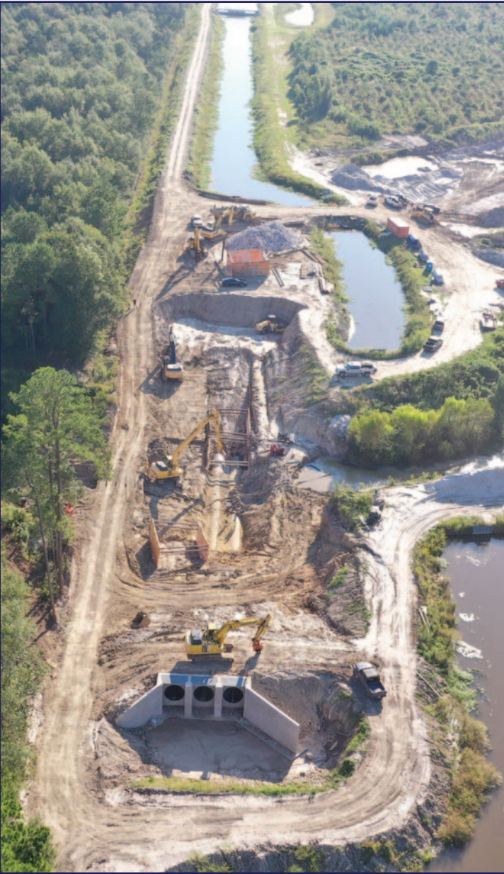
Claybar Siphon Project
