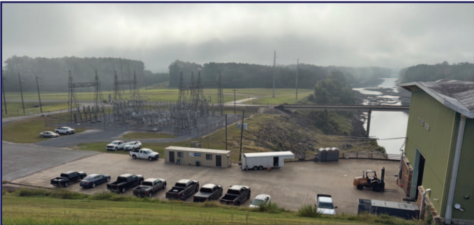
Toledo Bend Powerhouse
