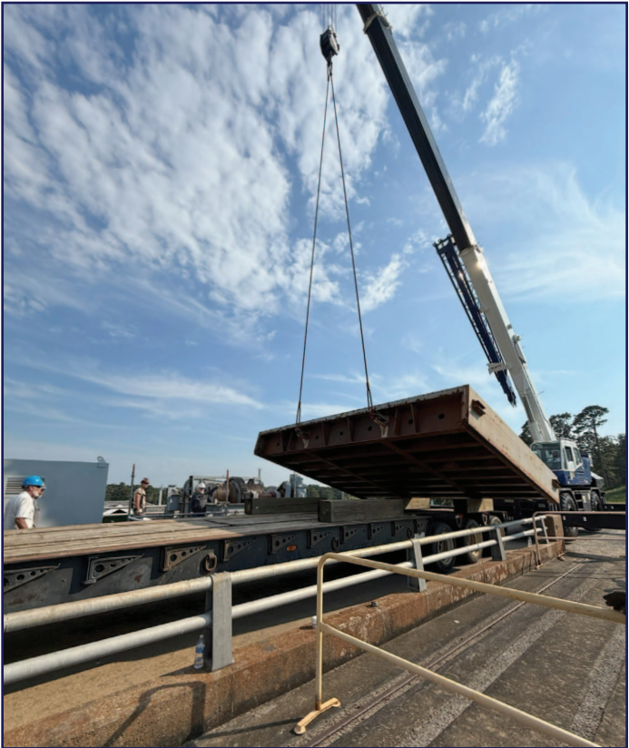
Powerhouse intake bulkhead installation
