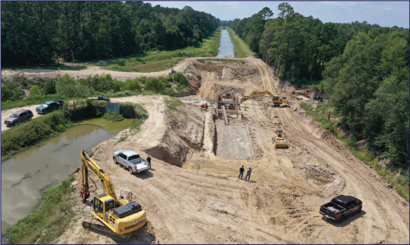
Claybar Siphon Project
