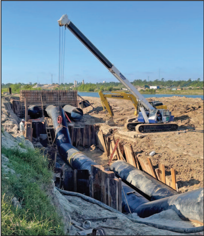
Womack Siphon Replacement Project
