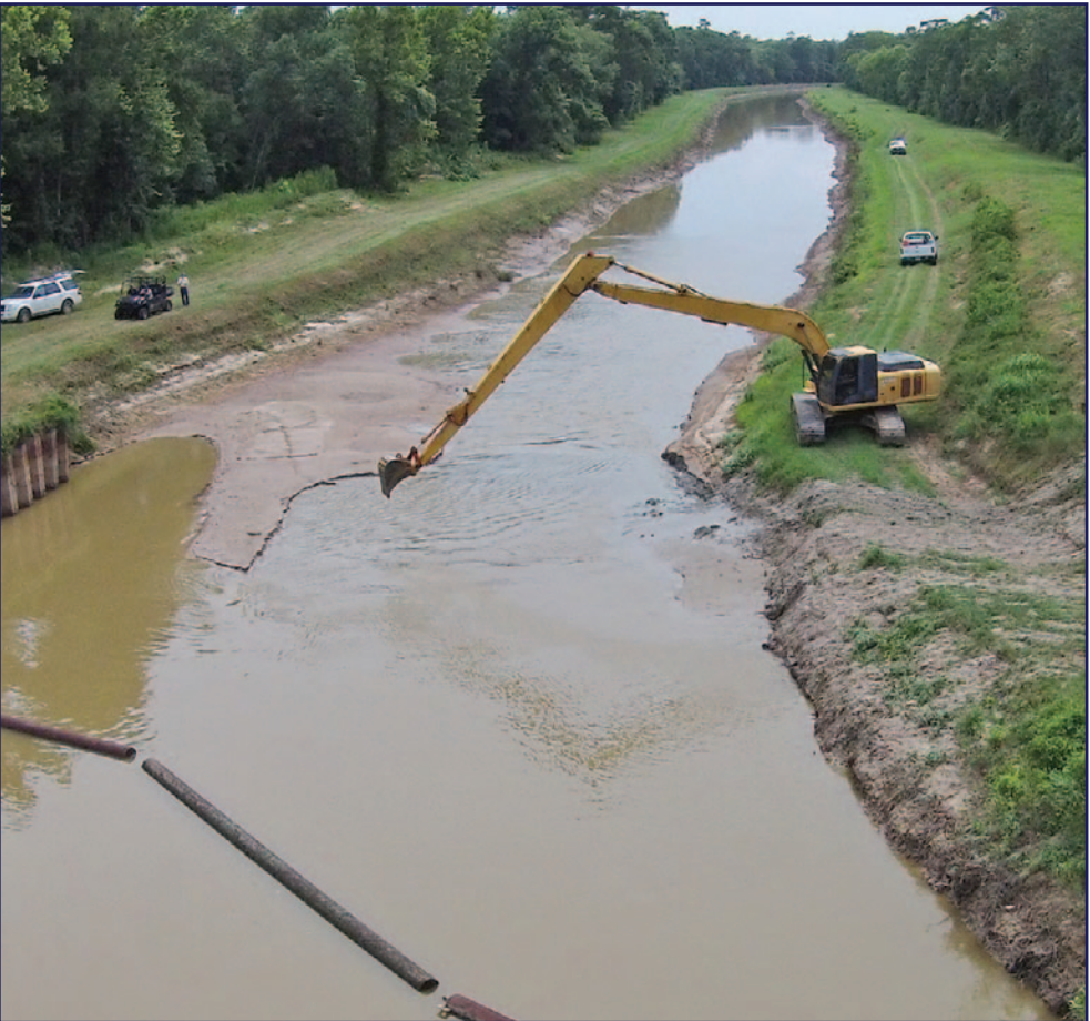
Removing accumulated silt
