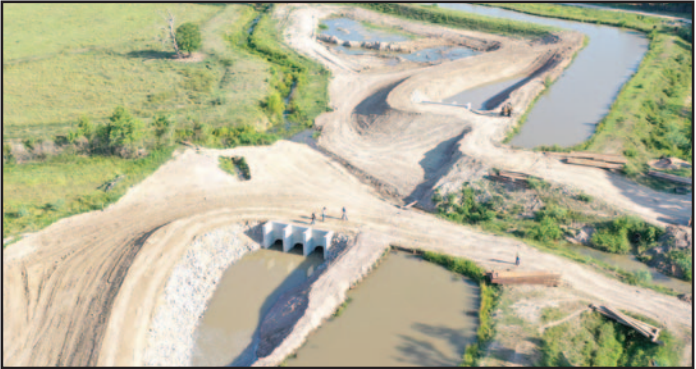
Womack Siphon Replacement Project
