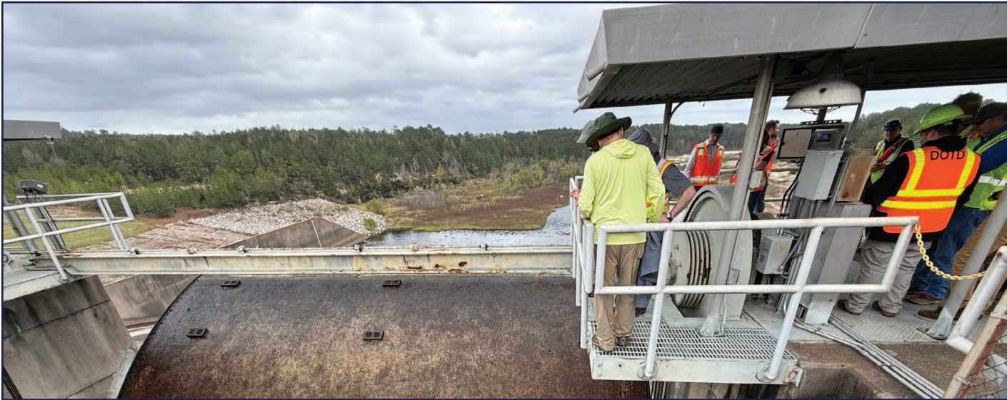
FERC Part 12D Inspection
