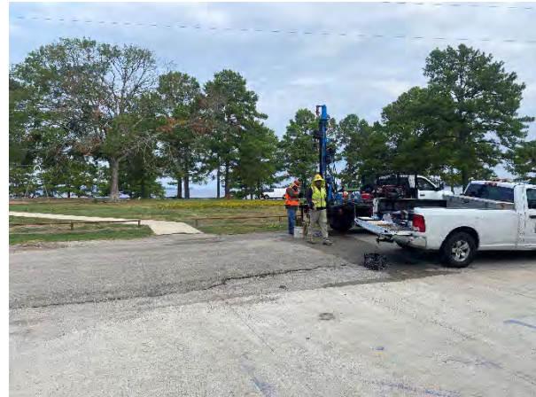
Facing North at Boring B-04
