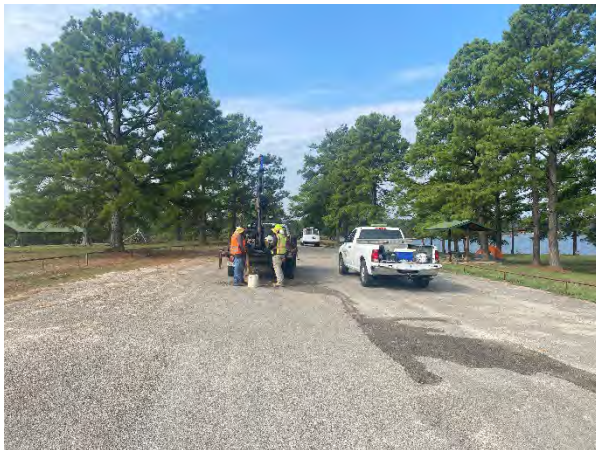
Facing Southwest at Boring B-07
