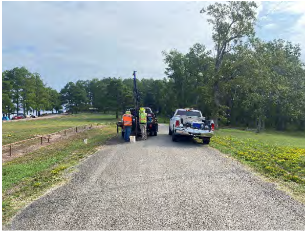
Facing Northeast at Boring B-05
