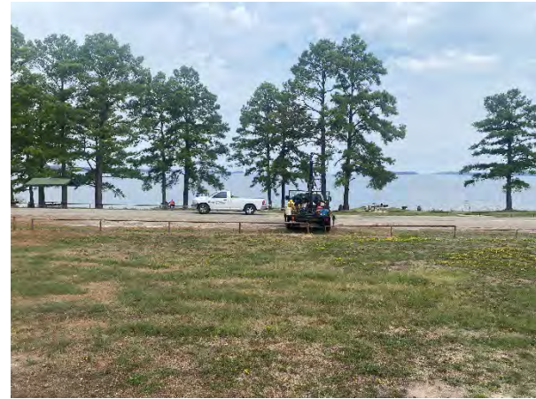
Facing Northwest at Boring B-06
