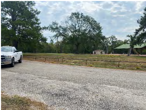
Asphalt Overlay Near Boring B-03
