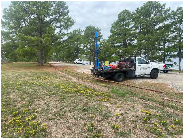
Distressed Pavement Near Boring B-06
