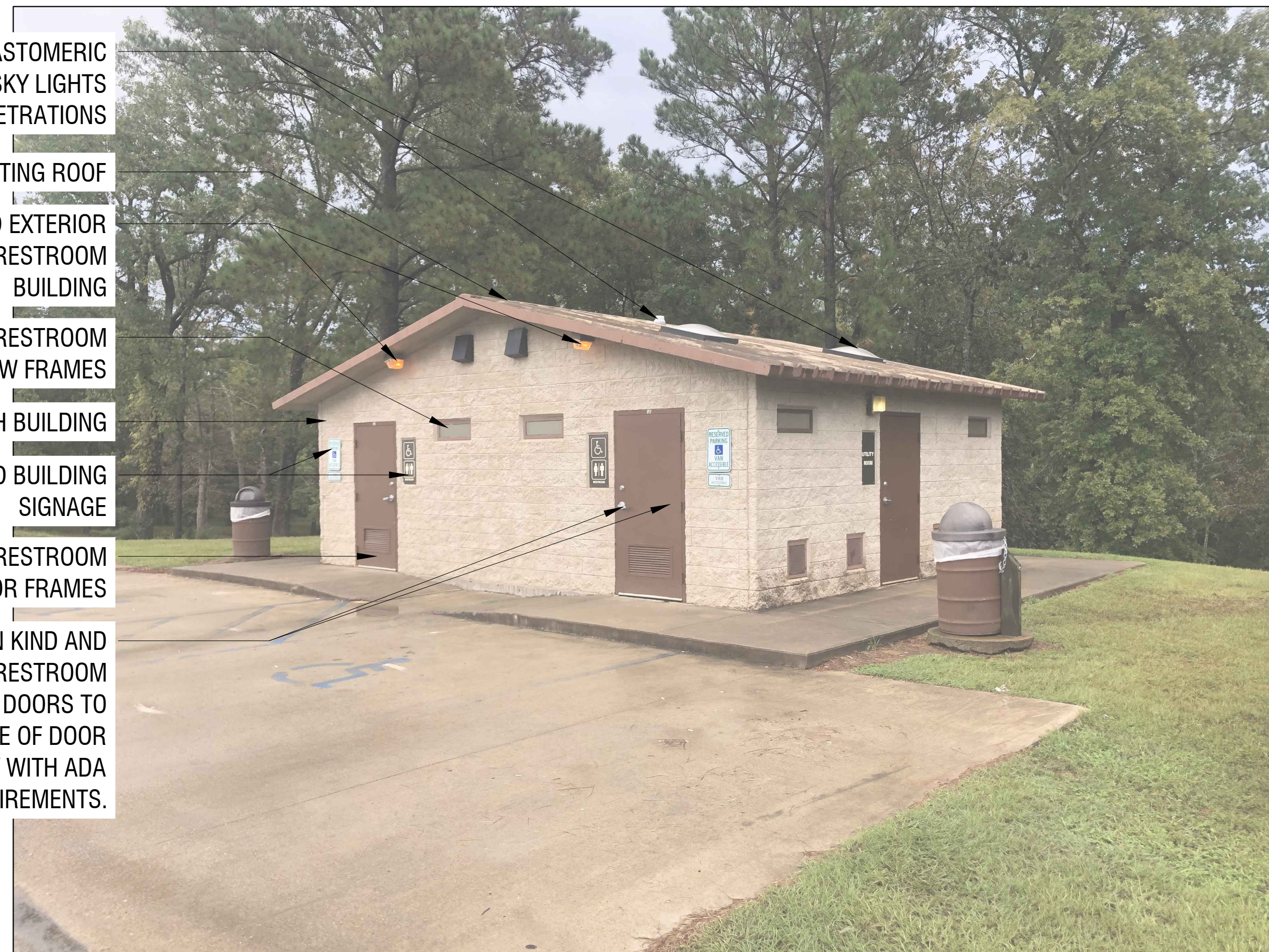
EXISTING RESTROOM RENOVATIONS
