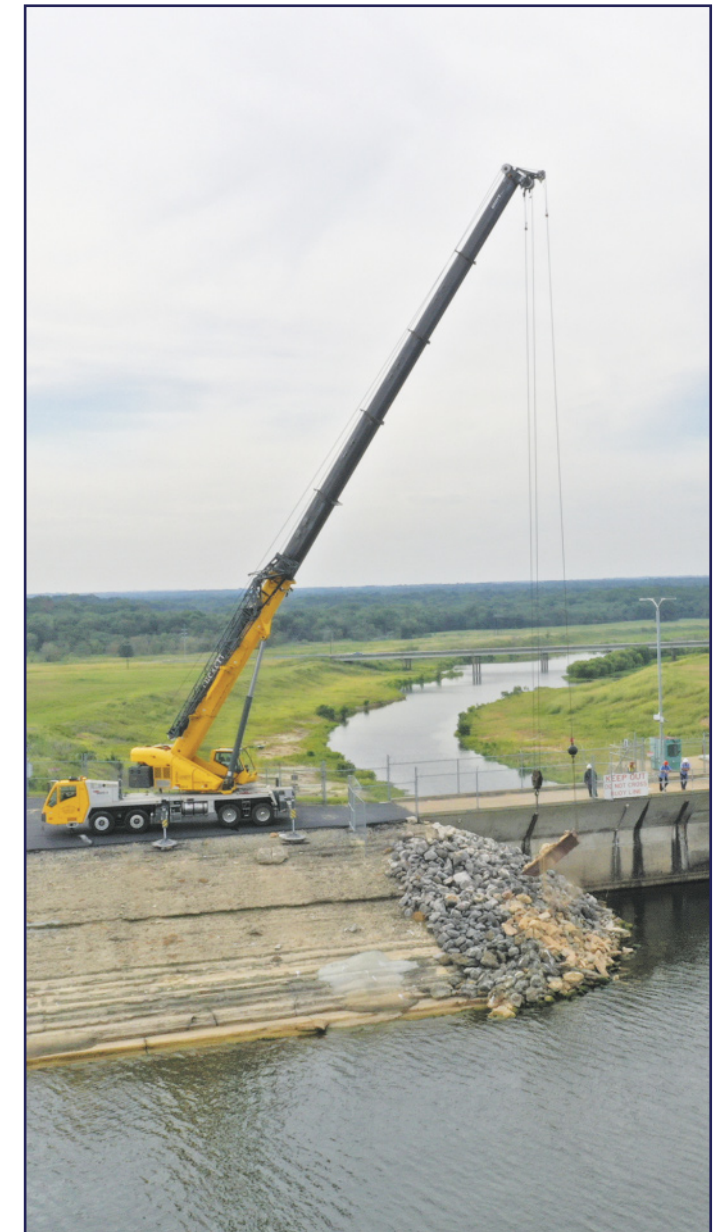
Riprap placement on wing walls
