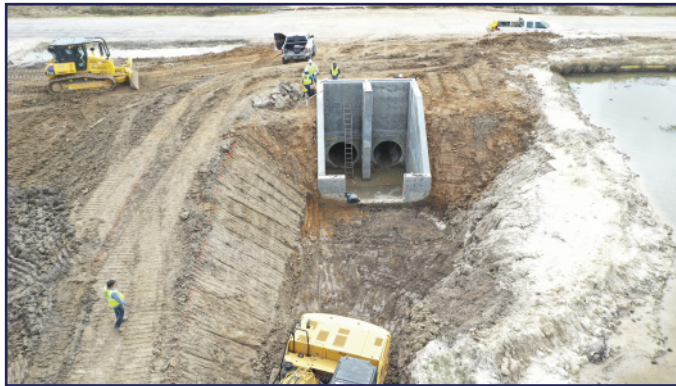
Tulane Road Siphon Replacement Project
