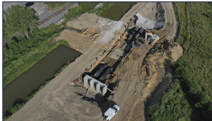
East Wynn Siphon Replacement Project
