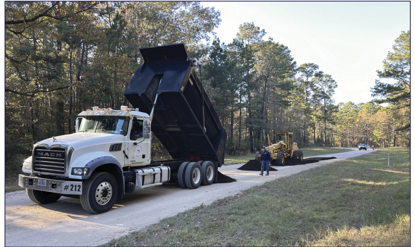
Road repairs at Haley's Ferry Recreation Area
