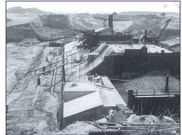
Lake Fork Dam construction
