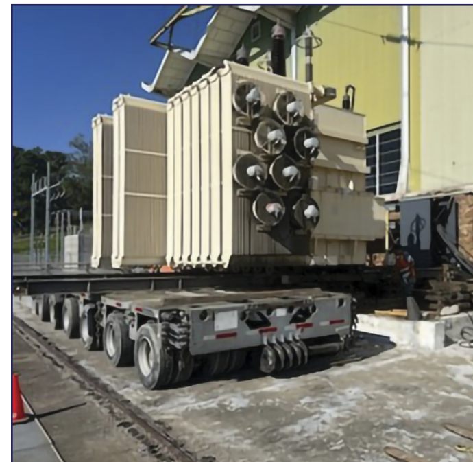
Removing old transformer
