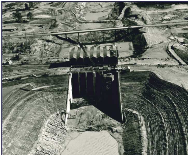
Toledo Bend Dam and Powerhouse construction
