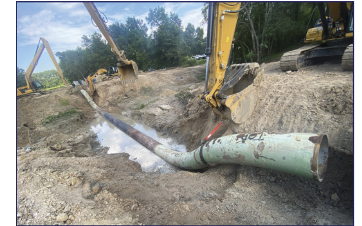
Cole Creek bypass siphon
