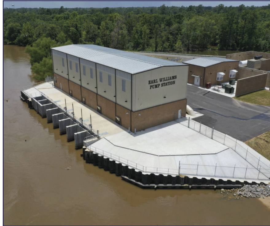
Earl Williams Pump Station
