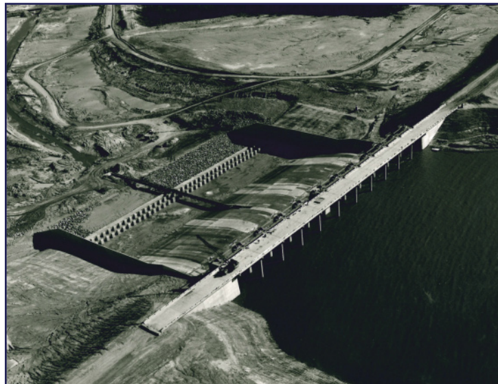
Toledo Bend Spillway construction
