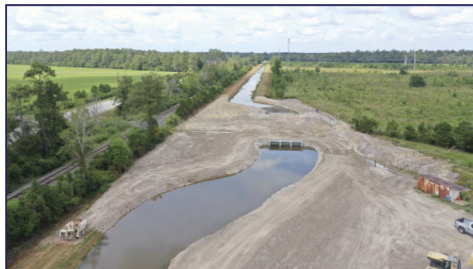
Completed East Wynn Siphon Project
