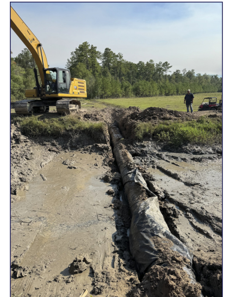
Main canal underdrain installation
