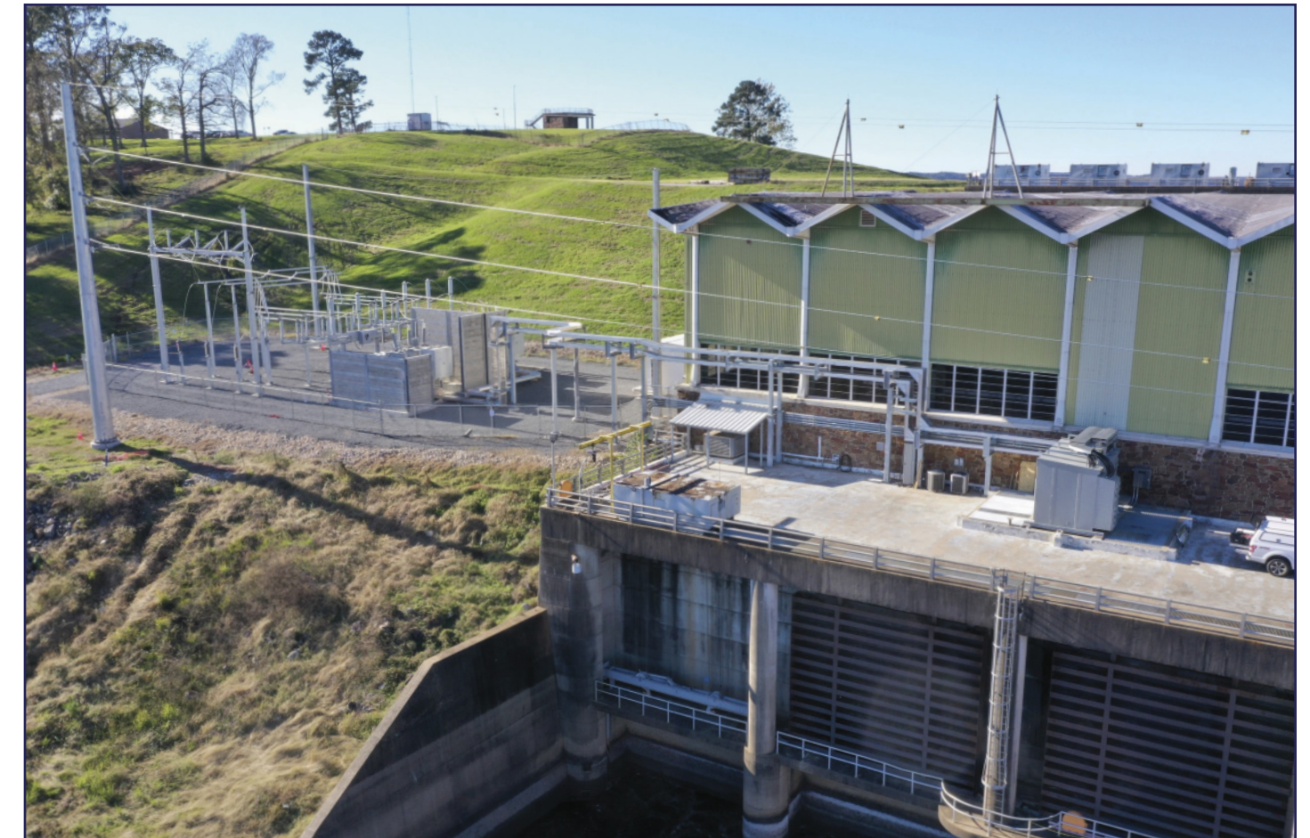
Substantial completion of the Generator Set-up Transformer Project
