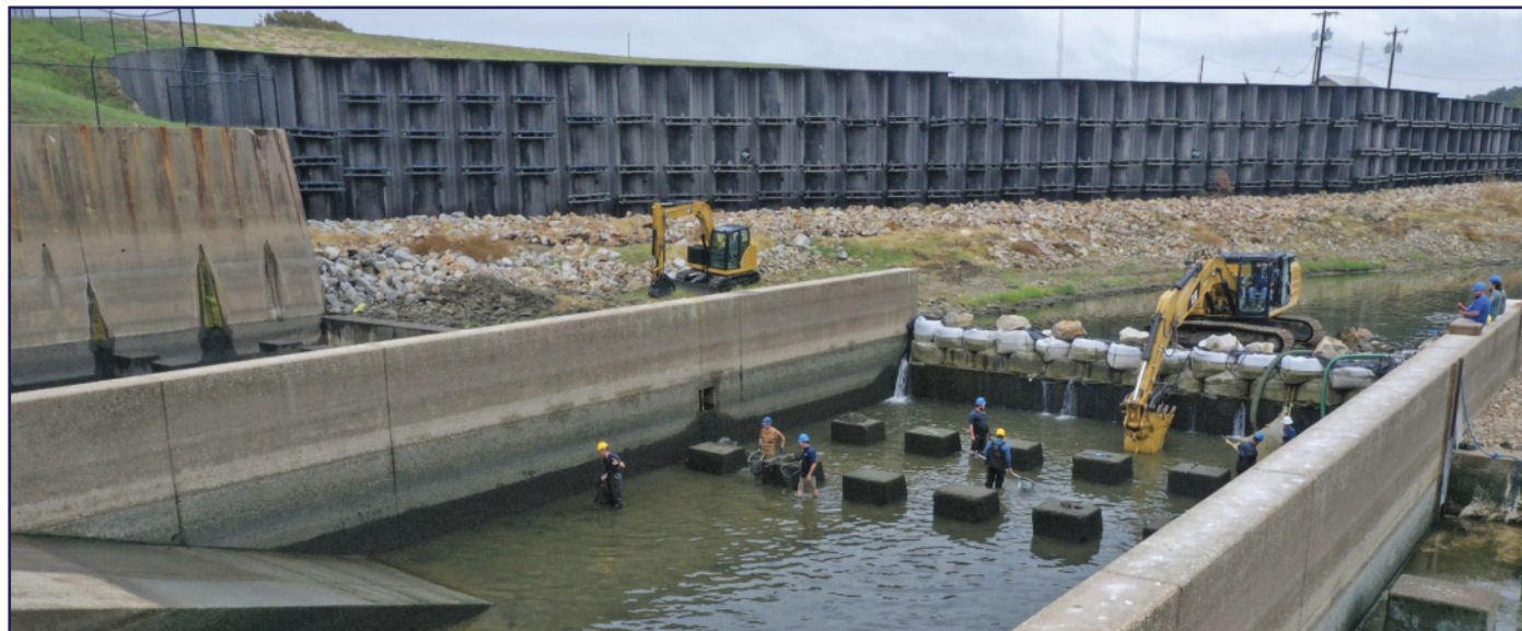
Dewatering of the stilling basin
